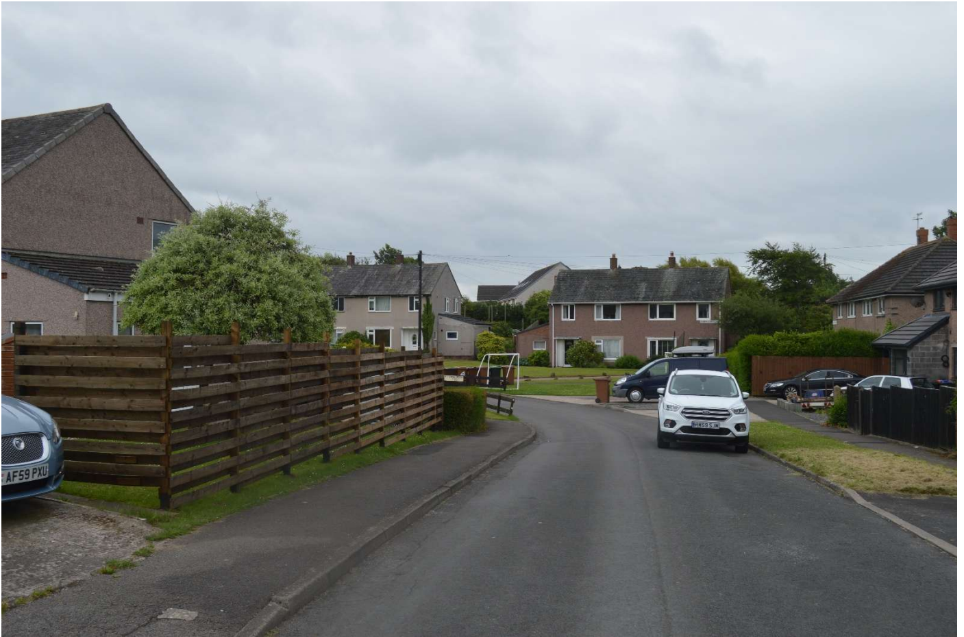
14 Example of timber fencing on the adjacent Fell View Road.
