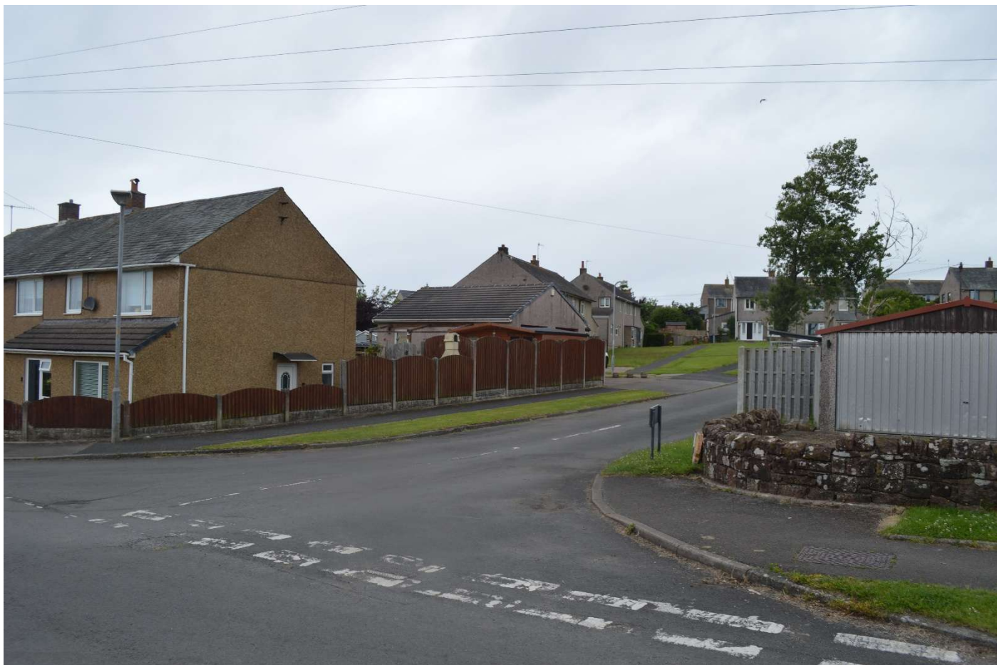
8 Existing garden fencing on Lingmell Crescent.
